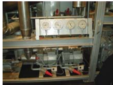
Bitzer Octagon-K compressors are used for the CO 2 cycle, the low stage in the cascade.
